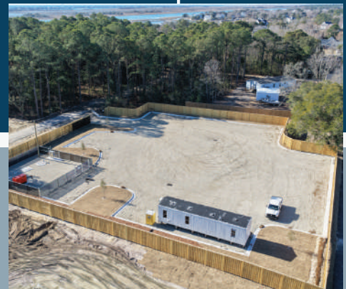
Boat Storage Area
